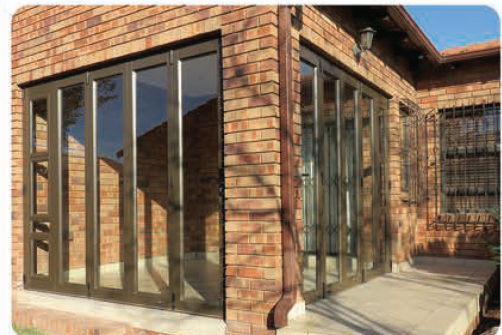
► After: Patio Enclosure Doors Closed
