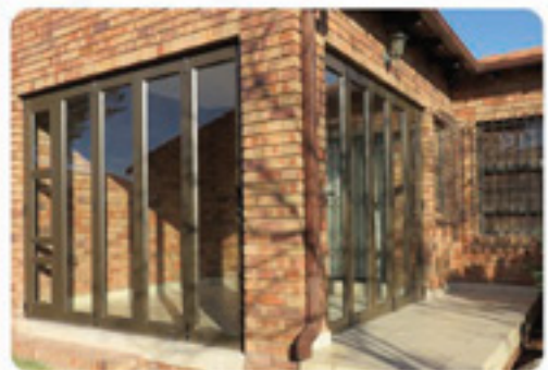
► After: Patio Enclosure Doors Closed
